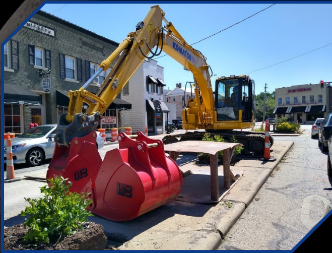
Heavy construction and excavation machinery.
